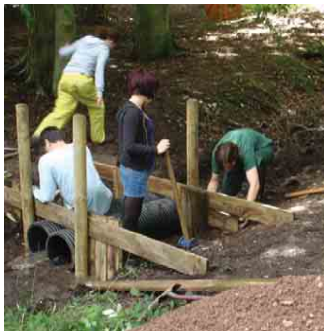
Volunteers build a culvert on Hazeley Heath
